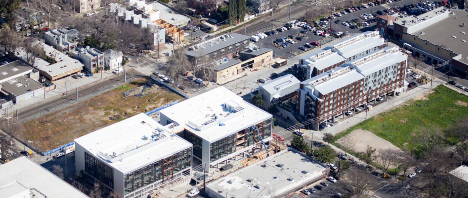
TOD PROJECTS UNDER CONSTRUCTION ALONG THE R STREET CORRIDOR IN SACRAMENTO
