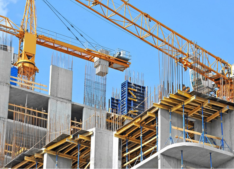
NEW CONSTRUCTION IN DOWNTOWN SACRAMENTO
