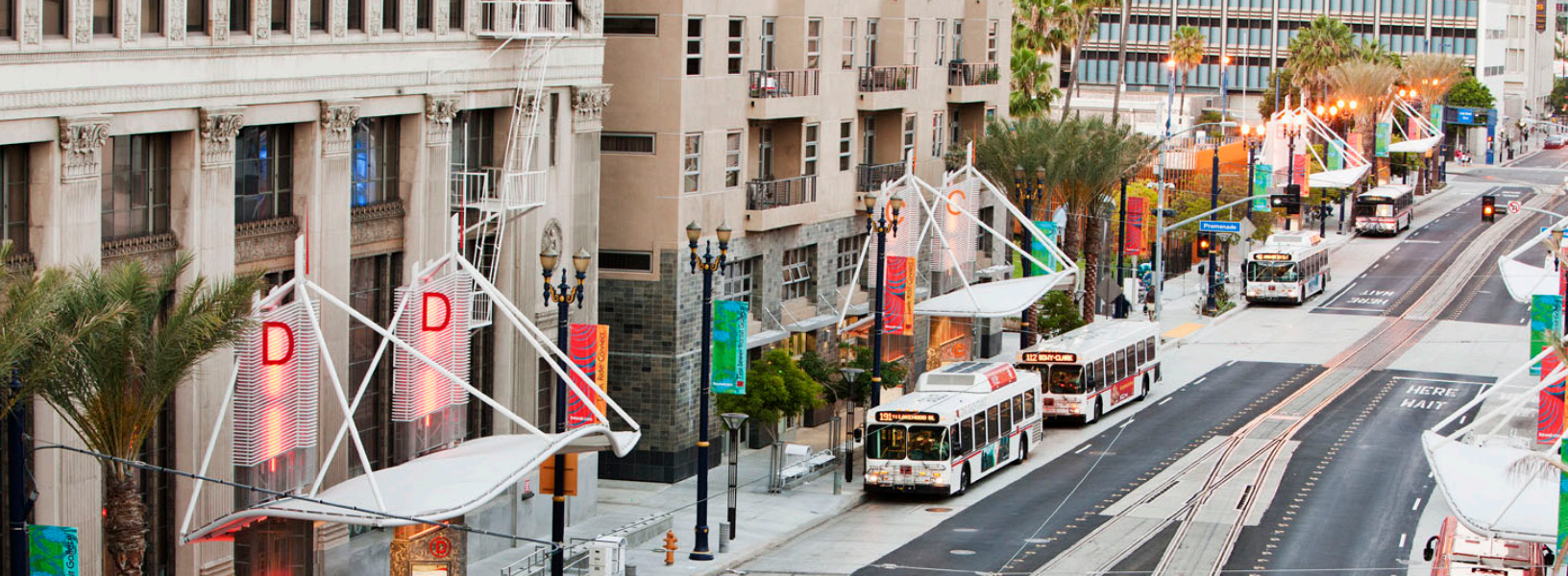
A MULTI-MODAL TRANSIT CENTER SURROUNDED BY TOD
