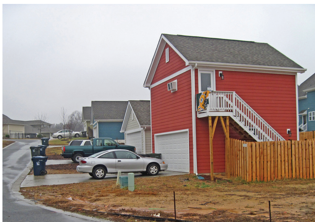
Figure 5.9. Accessory dwelling unit above a garage in Huntersville, North Carolina (Flickr photo/Brett VA (CC BY 2.0))
