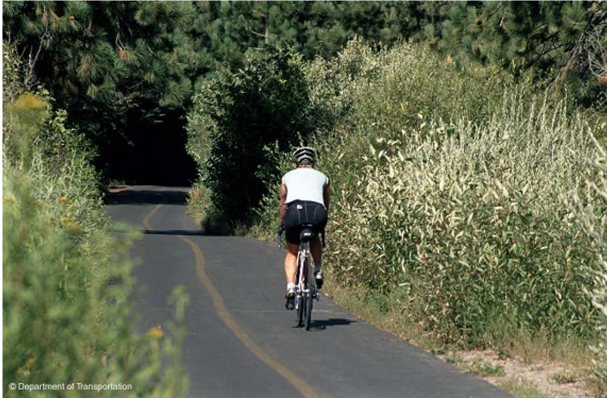
Part of the 32-Mile Long American River Bike Trail
