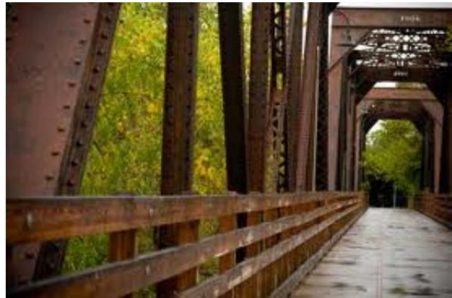
Train trestle in Winters
