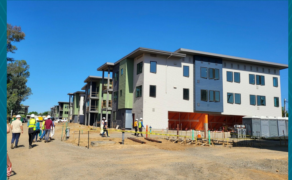
San Juan apartments on Stockton Blvd. (Green Means Go underground infrastructure project, City of Sacramento)
