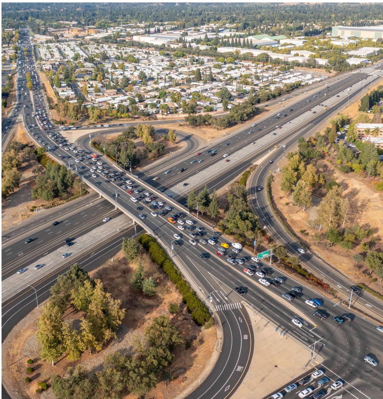
The US 50/Sunrise Boulevard Interchange provides access to Rancho Cordova's employment centers, commercial districts, and recreation along the American River Parkway.
