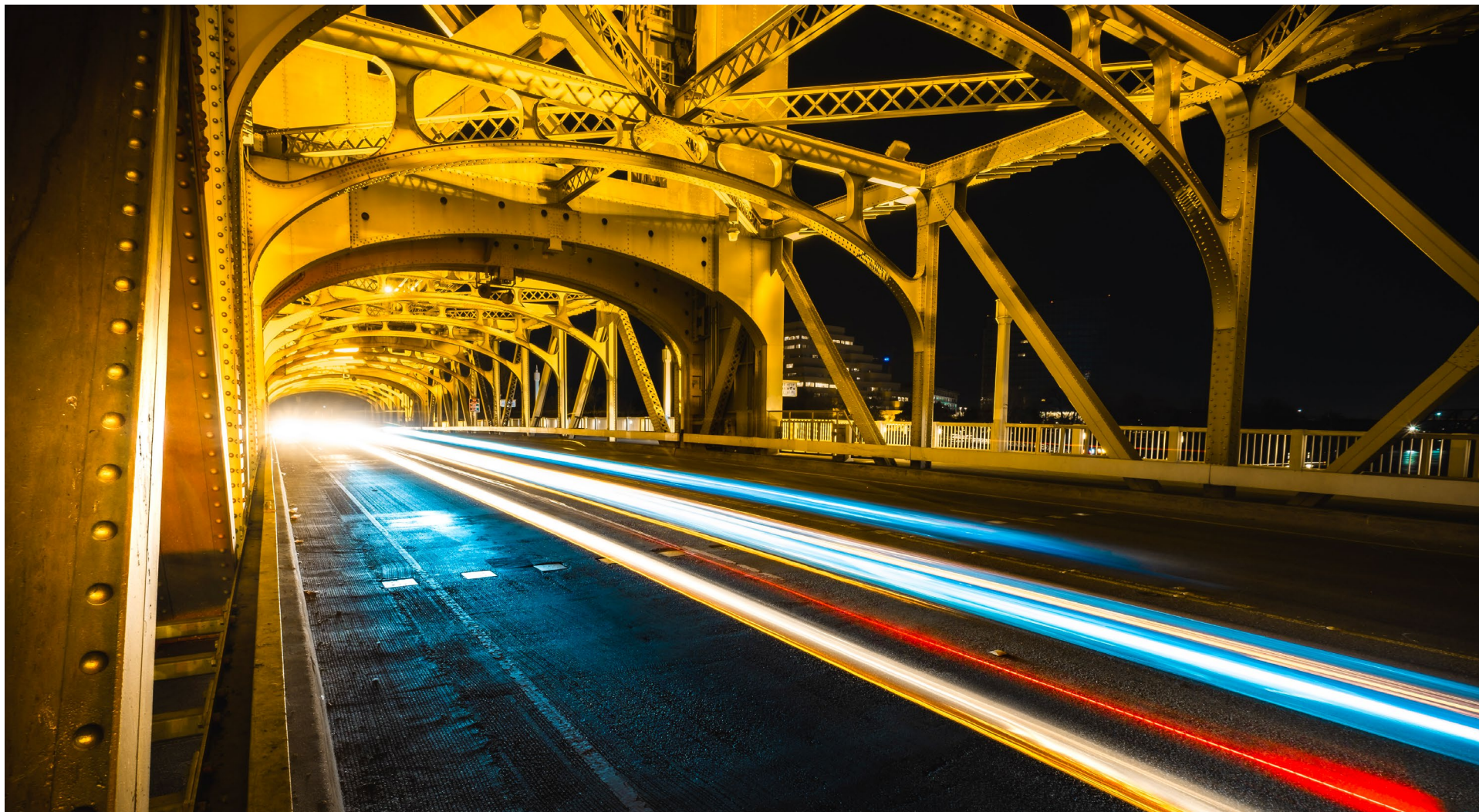
The Tower Bridge is a critical link between Sacramento and West Sacramento, supporting thousands of daily vehicle, bicycle, and pedestrian trips.
