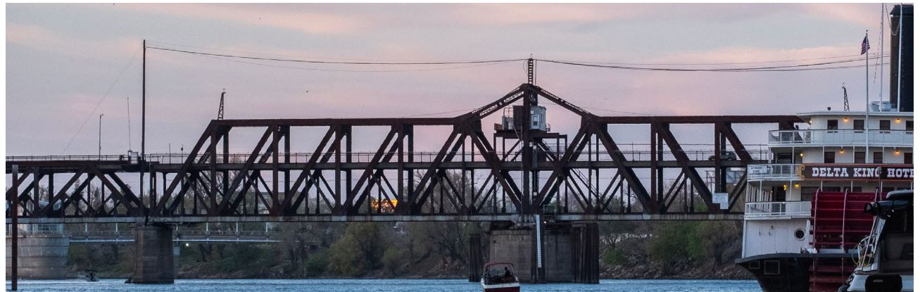
The historic I Street Bridge serves as a key connection between the Cities of Sacramento and West Sacramento.
