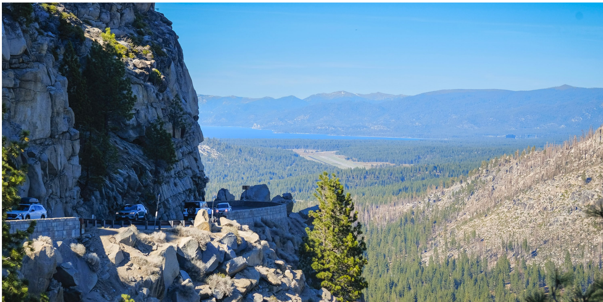
US 50 serves as a critical travel route for Sierra communities and to access Lake Tahoe.
